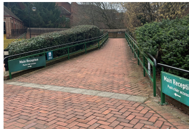
CIVIC CENTRE RAMPED APPROACH
